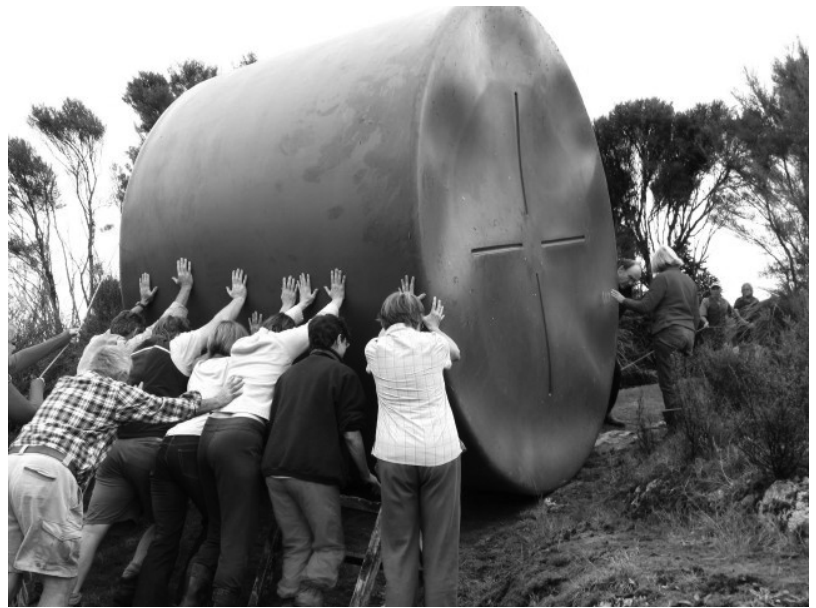
Team work at Mangarakau – pushing the water tank into place
