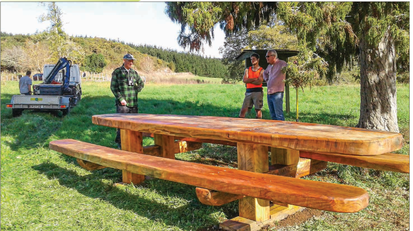
Installation of the new picnic table. (Photographs by Sharen Graham)
